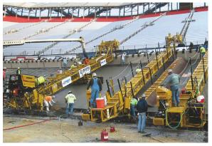
Baker Concrete Construction, Monroe, Ohio, paves the .533-mile, high-banked oval racetrack at Bristol Motor Speedway.
