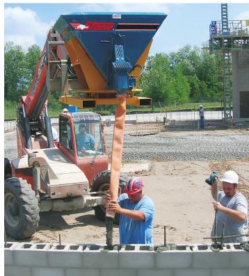
Groutzilla and its 20-cubic-foot hopper locks on the forks of a telehandler or forklift. It is powered by the forklift's auxiliary hydraulic circuits.
